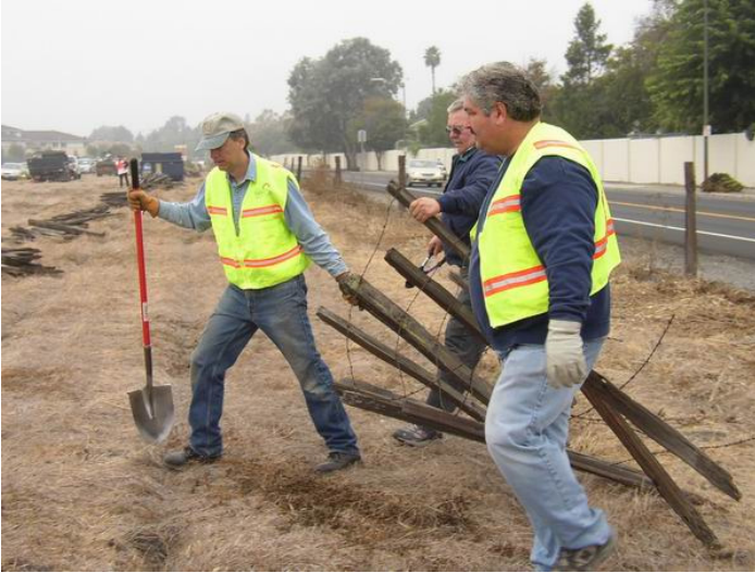
Hauling a Fence Section Away
