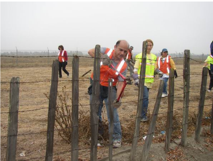
Cutting The Fence Into Sections
